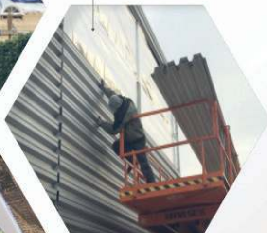
Airflex® Permovap15, dampopen, achter wandbeplating.
