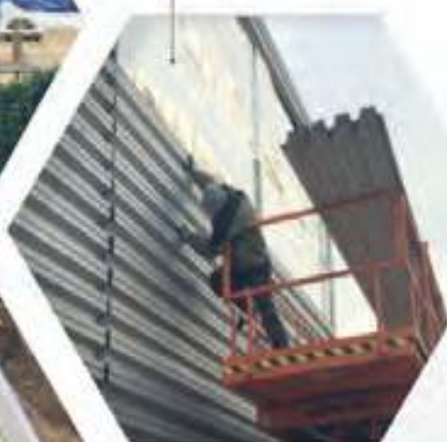
Airflex® Permopak S, dampopen, achter wandbeplating.
