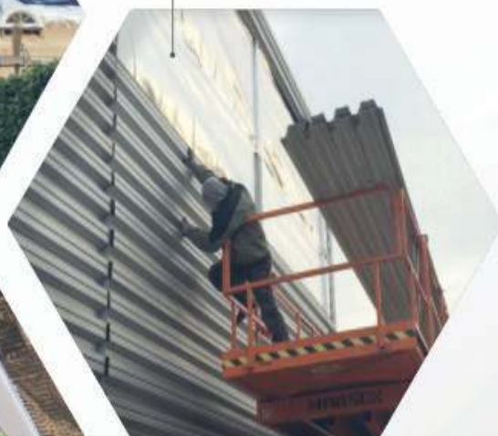
Airflex® Permopak15, dampopen, achter wandbeplating.
